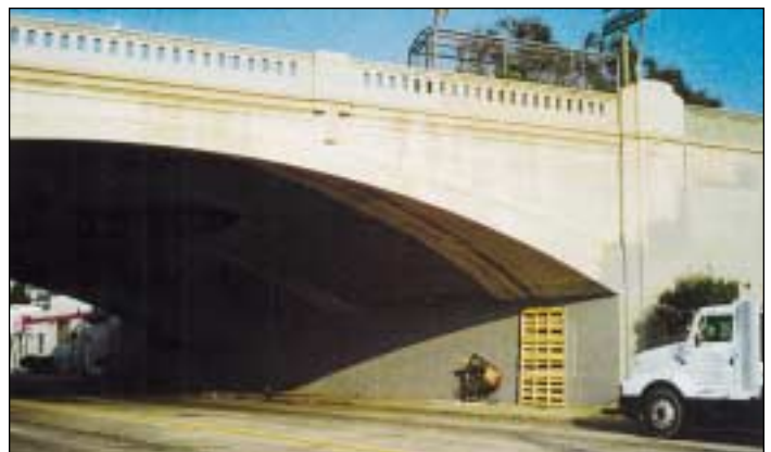
Entrance to stairway tunnel and chainlink cage above.
