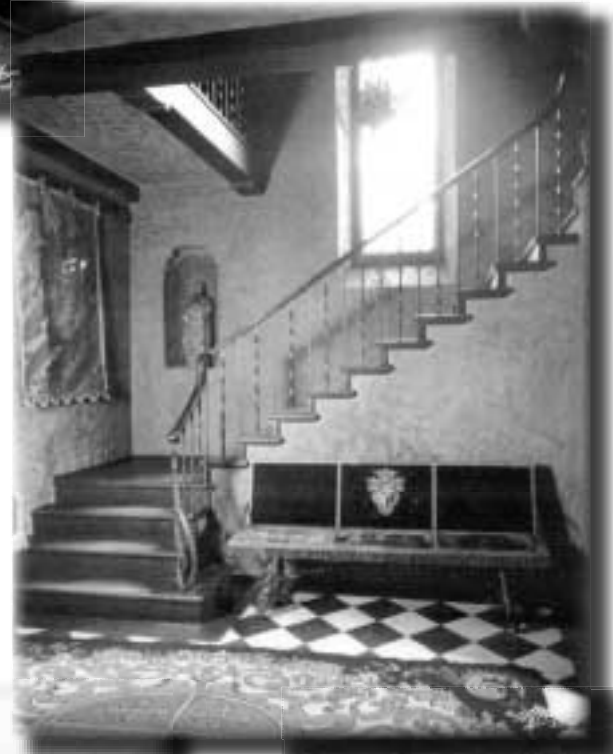
The entry hall
